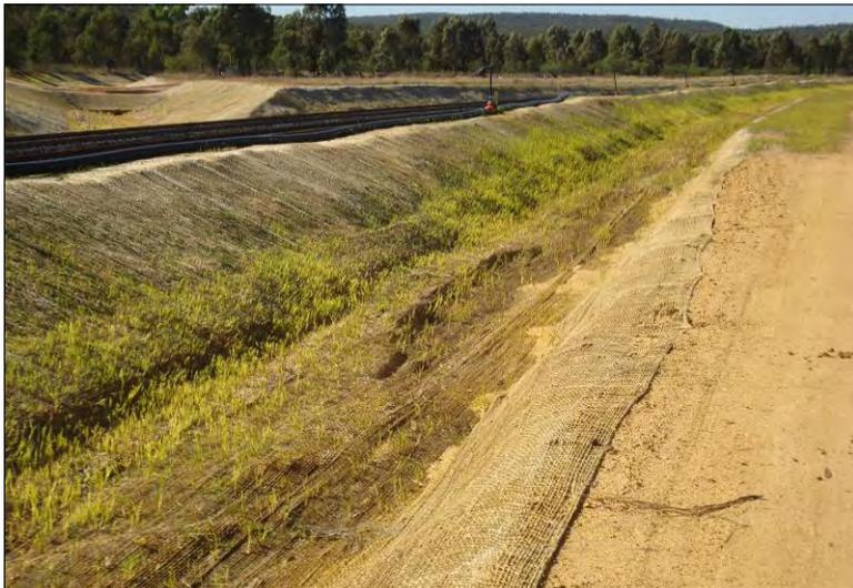
Photo 19: Soil Stabilisation works near Rail Loop (May 2010)
