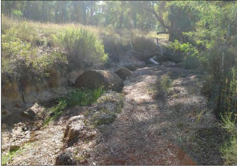
Photo 17: Hay Bales installed in Bora Creek (May 2010)
