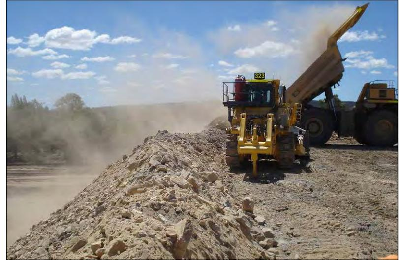
Photo 6: Construction of Environmental Bund (Dec 09)
