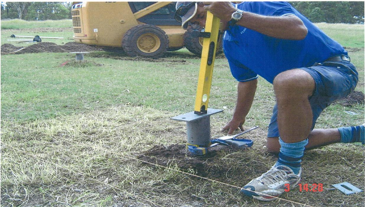
3) Tek screw fix pier cap to screw pier using 14# x 30mm tek screws.
