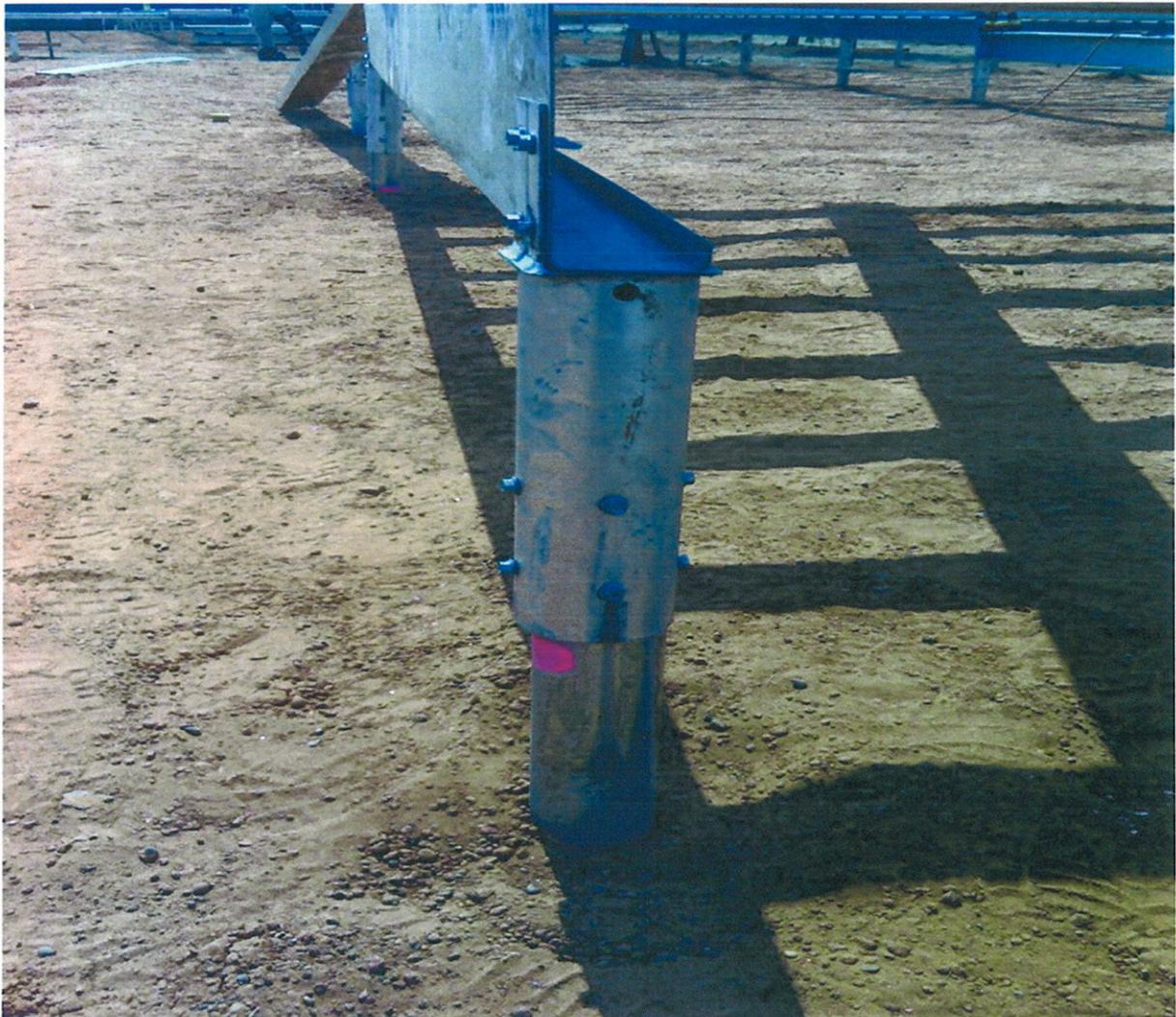
**Series 1 Screw Piers installed and fastened to Lysaght "C" section.**
