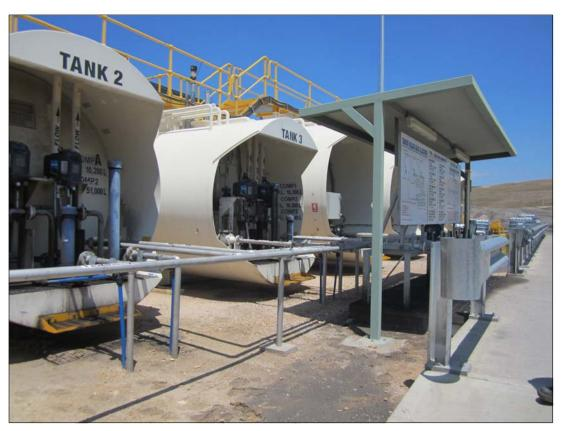
PLATE 6 Fuel tanks at Open Cut Workshop - tanks double skinned and fill points enclosed by drive-over bunds
