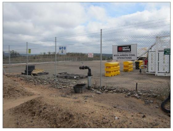
PLATE 3 Diesel fill point at Downer Blast Services compound - note no secondary containment
