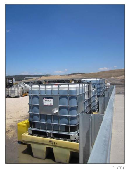
TLATE 6 1000L mini-bulk containers on bunded pallet - note no secondary containment from toppling or leaks under pressure
