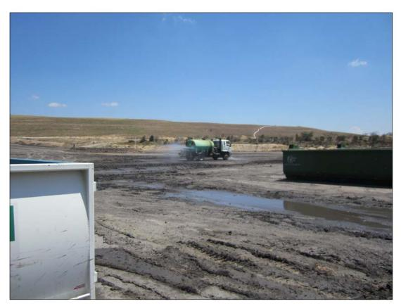
PLATE 4 Water cart in operation around Open Cut Workshop
