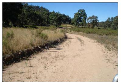
Photo 25: Stage 2 Area – Murragamba Valley showing grading of access track (May 2010)
