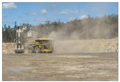
Photo 13: Excavation of dry soil layer and overburden (Dec 09)
