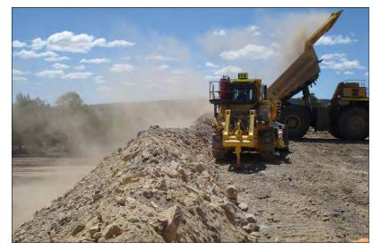
Photo 6: Construction of Environmental Bund (Dec 09)
