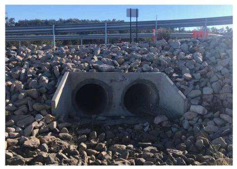
Figure 2-2 - Example of Proposed Culvert C23
