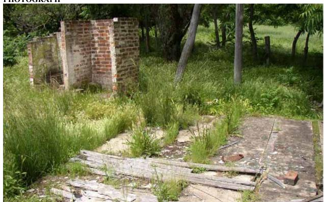
P008 Showing east room with timber floor over concrete plus fireplaces
